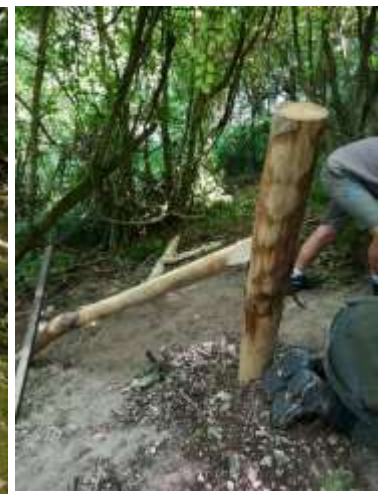
Figures 4a & 4b: Fence post being installed
